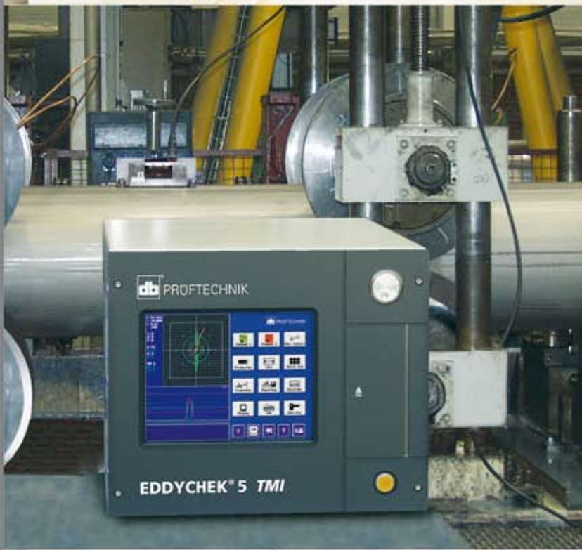
Typical installation in calibration section of a tube mill
